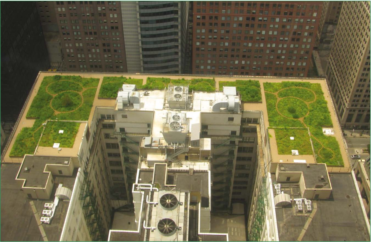
The greened roof of the Chicago City Hall.
