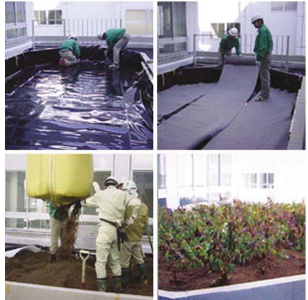
Built-in Place Installation of a rooftop garden
