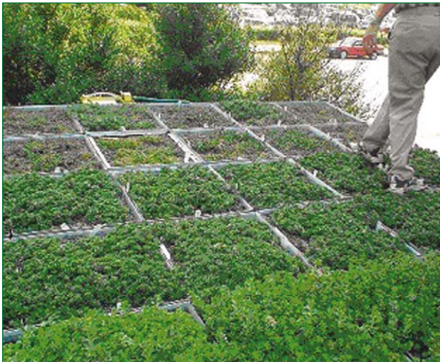
Modular Installation of a rooftop garden
